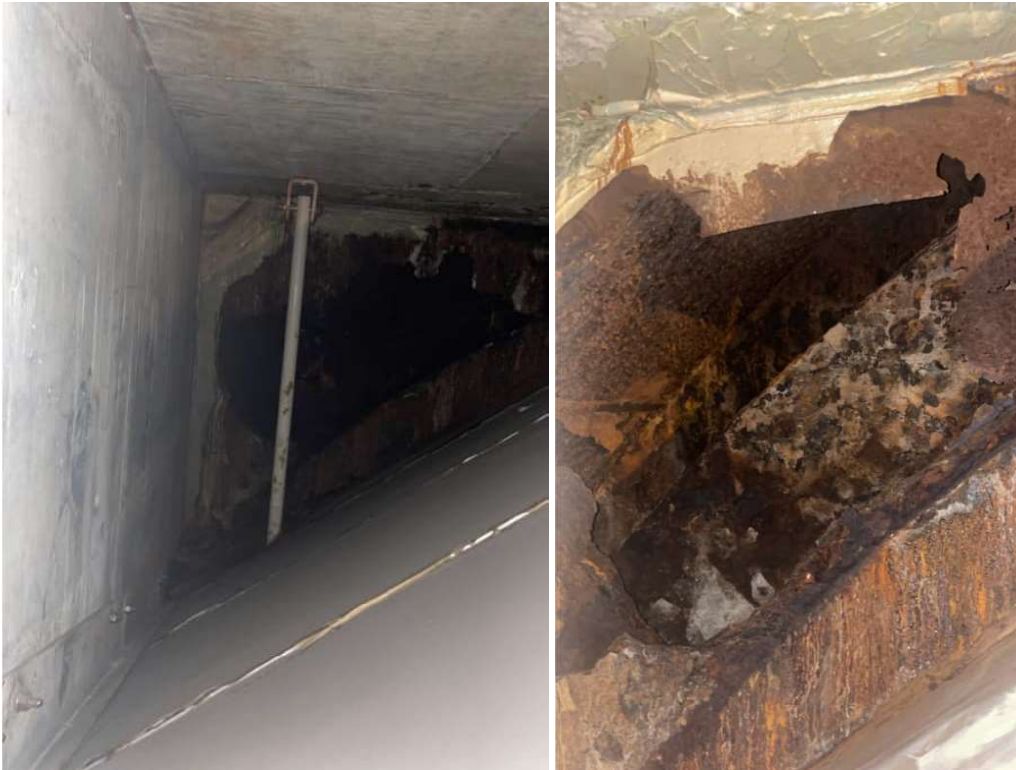
Figure 6: MMBT Exhaust Duct Damage from Leak/Access to Void
