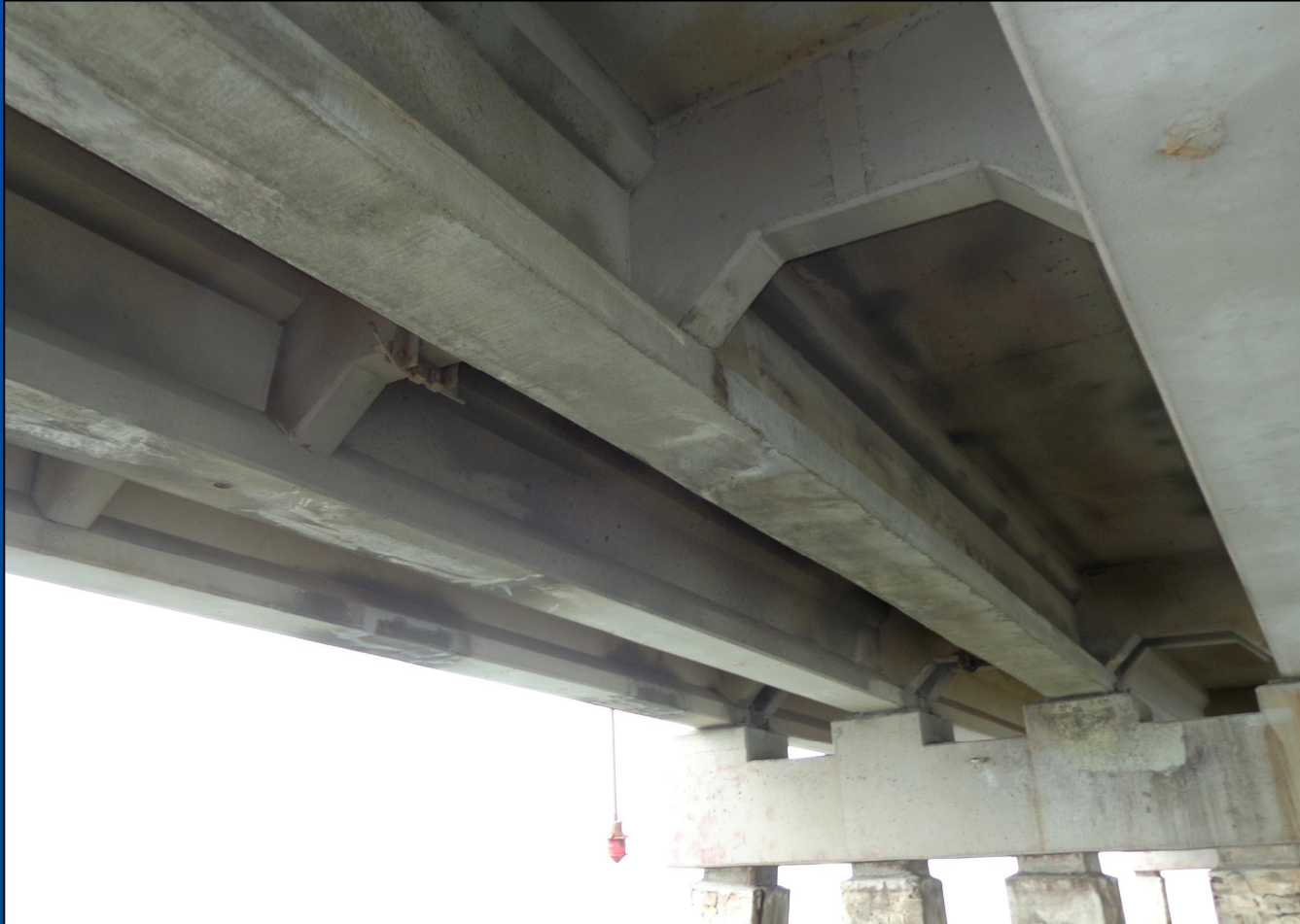
Span 56, Beam 5 – After Patching
