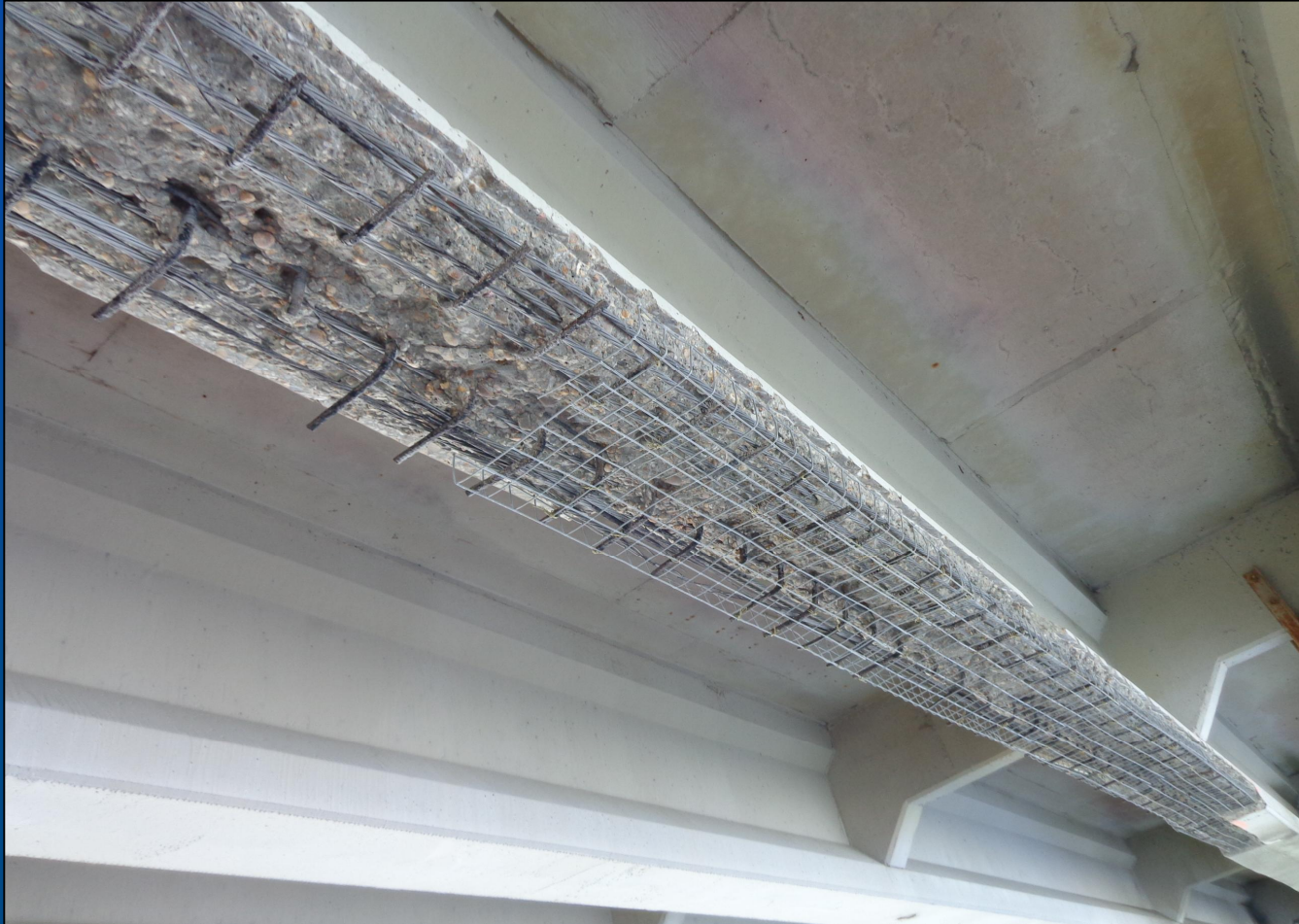
Span 56, Beam 5 – During Patching
