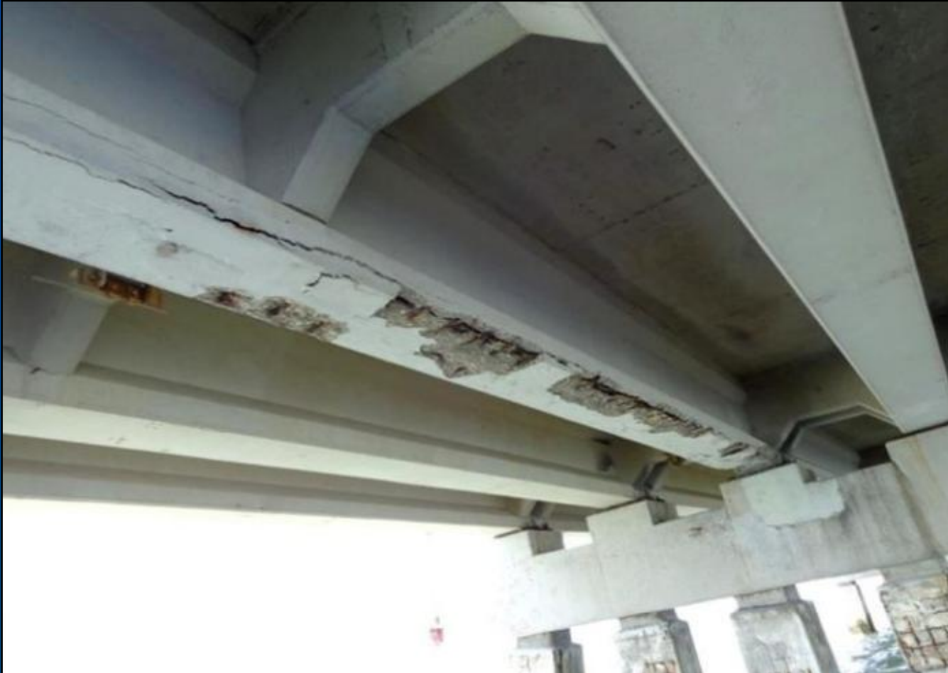
Span 56, Beam 5 – Before Patching
