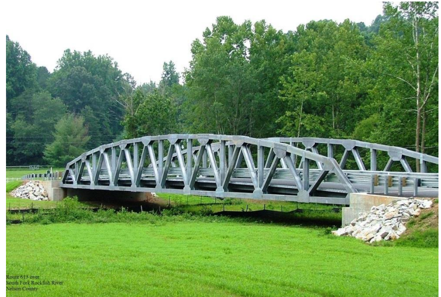
Example: US Bridge Cambridge Truss
