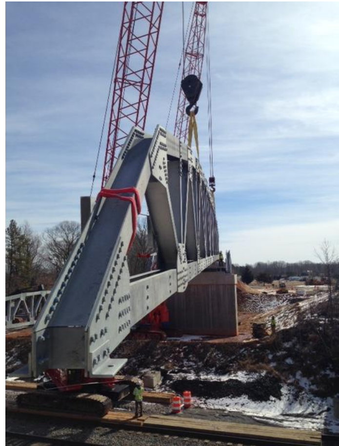
Example: US Bridge Cambridge Truss, all bolted
